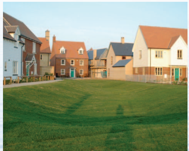
Infiltration basin in dry state, Ipswich
