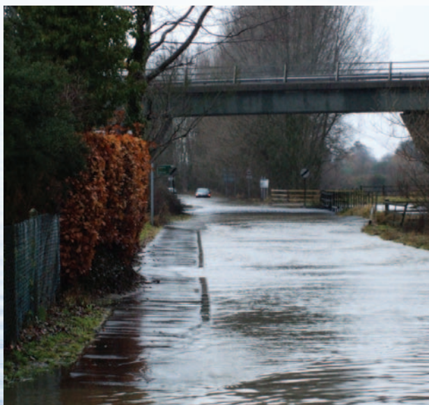
Highway flooding in Beyton in 2009. Work has now taken place to alleviate this problem
