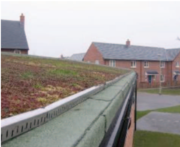
Green roof on a shed
