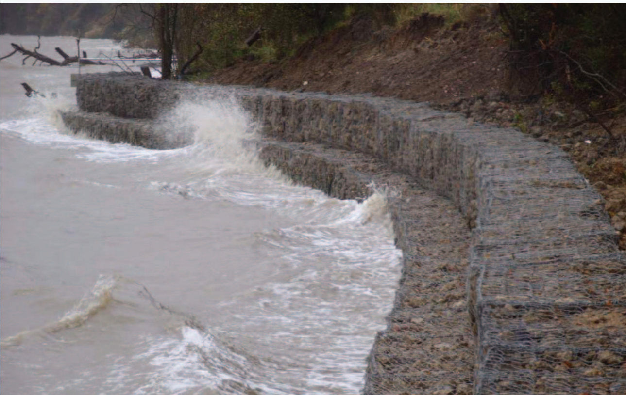
Coastal Erosion protection at Shotley
