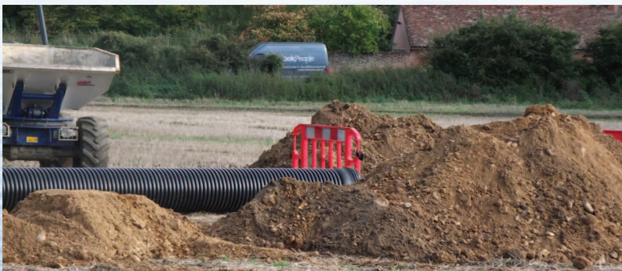
Below: Putting in new drainage pipe in Long Melford
