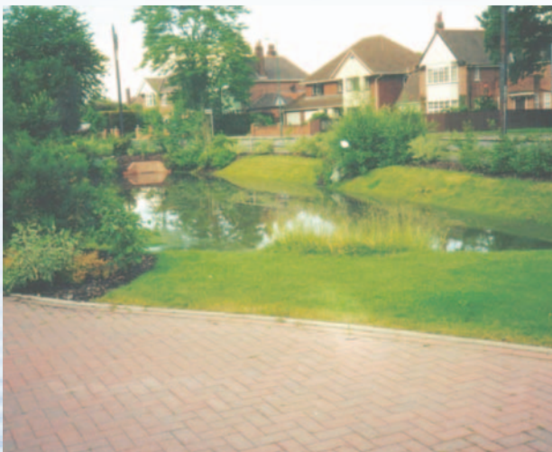
Detention Basin, Ipswich
