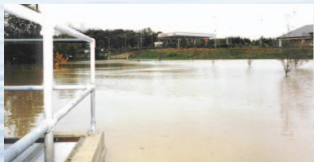
Coreys Mill Water Meadow, Stevenage Flooded state
