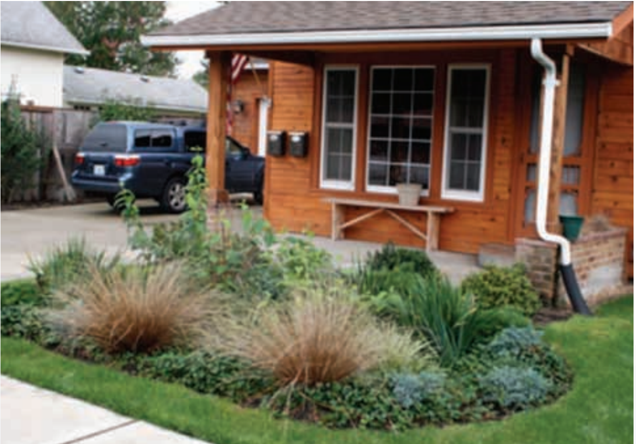
Typical rain garden taking water off the roof
