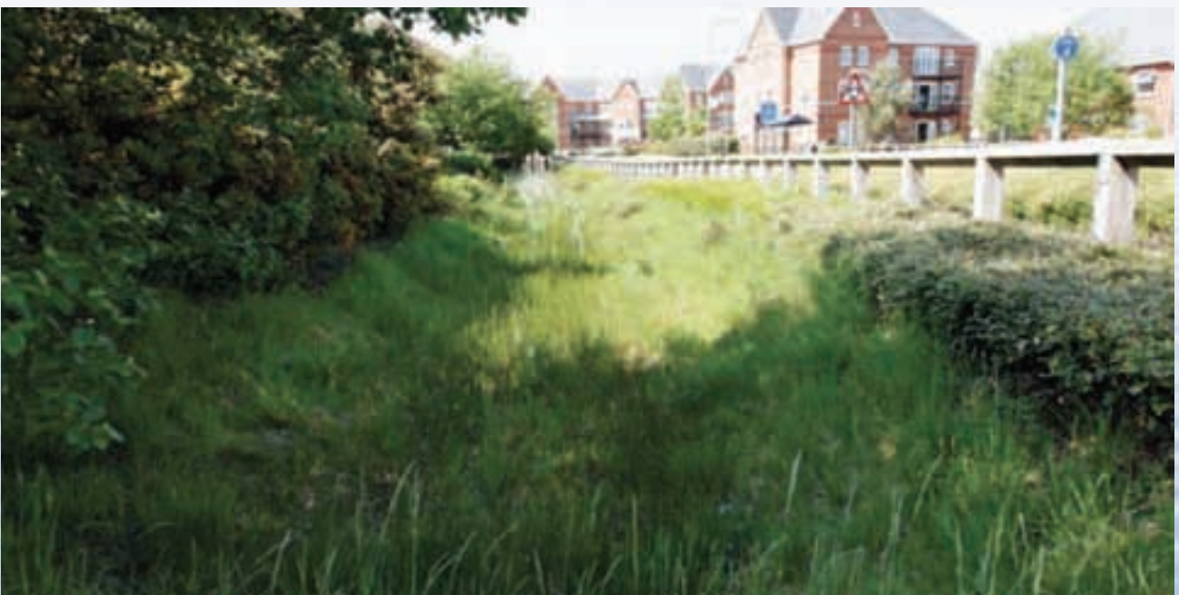
Sustainable drainage alongside a highway
