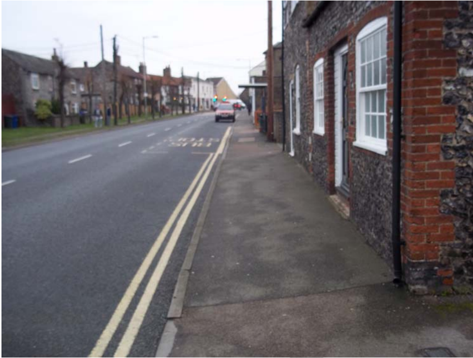
Photograph 3 – London Road looking towards the junction with the High Street
