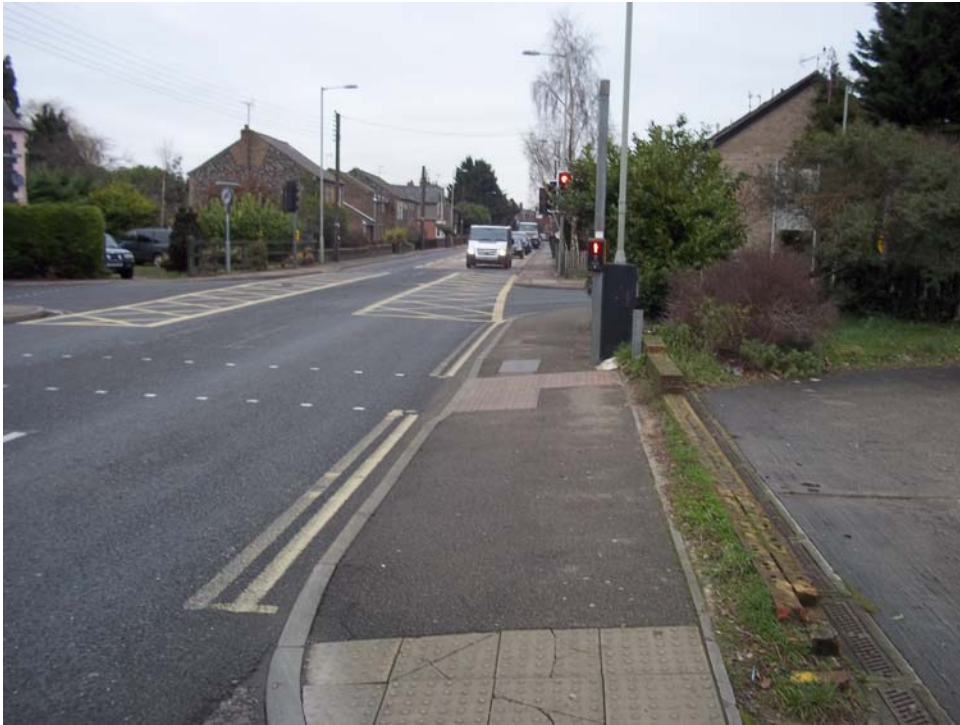
Photograph 1 – London Road looking towards the junction with Church Road/Rattlers Road
