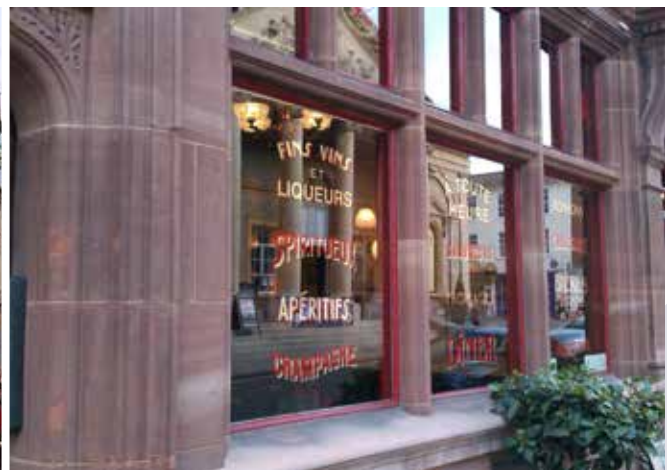
Gilded paint window lettering in an appropriate size and style for the building
