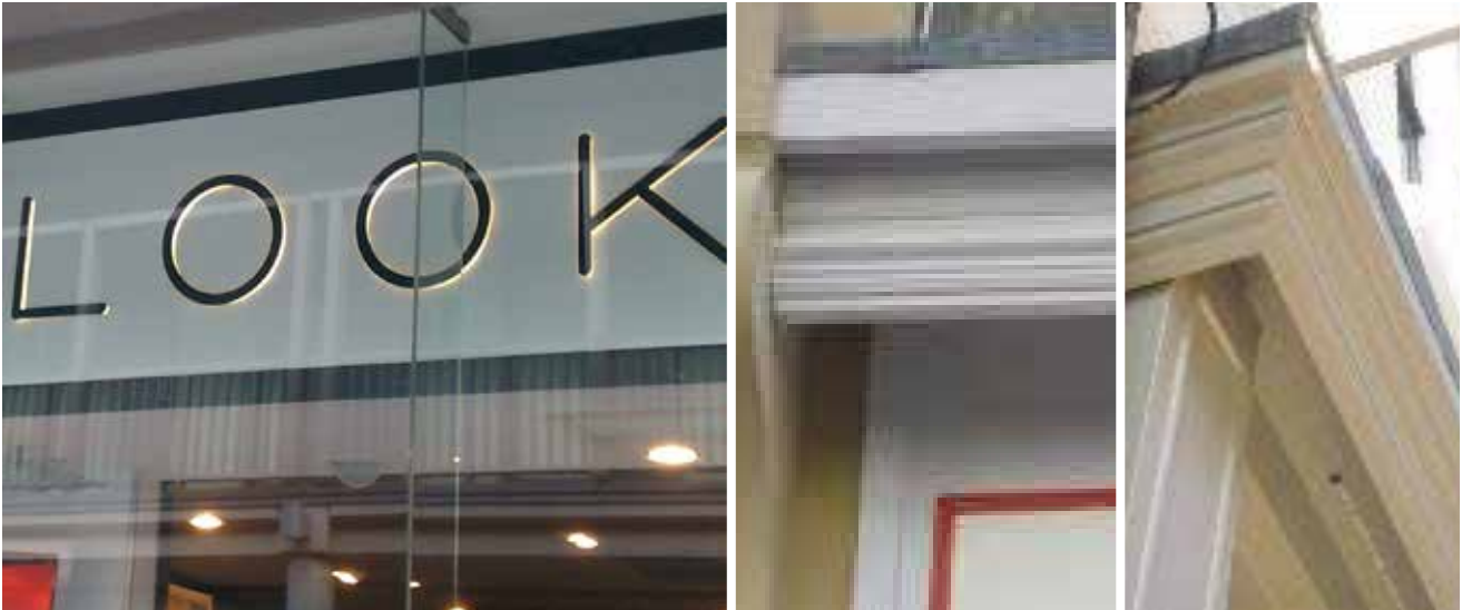
Example of halo style lighting
