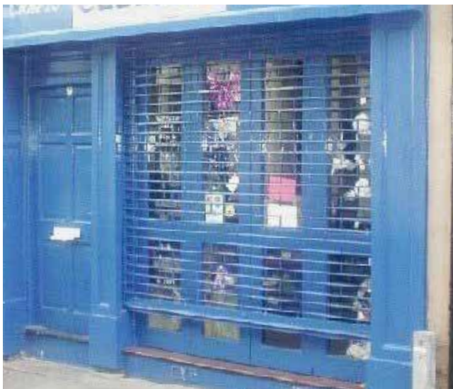
External brick bond lattice roller shutter with housing concealed in the fascia
