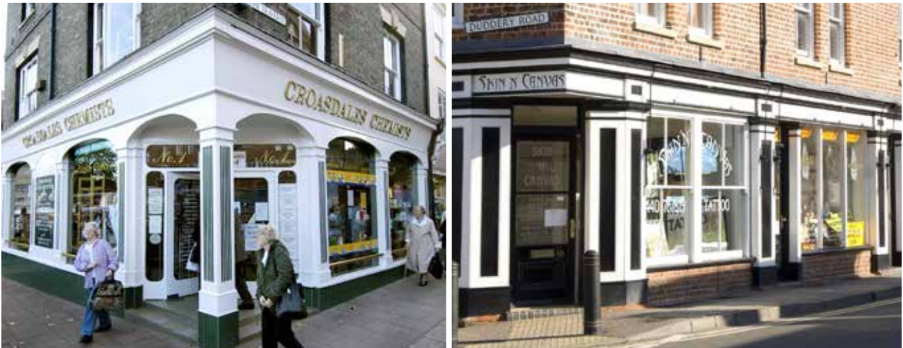
Examples of shop fronts incorporating the basic elements of good shop front design and quality materials
