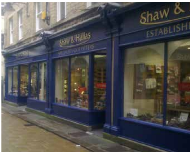
Contemporary stall riser
