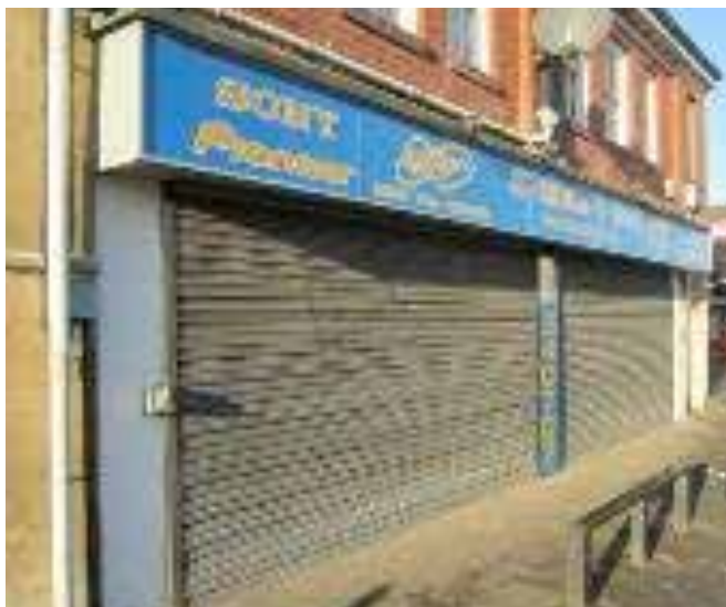
Visually harsh and unsympathetic external roller security shutters with bulky grille boxes
