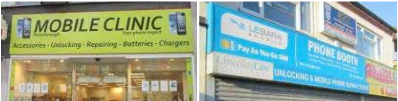
Inappropriate oversized fascias and deep projecting box fascias
