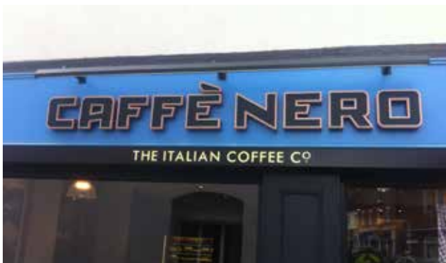
Contemporary style fascia
