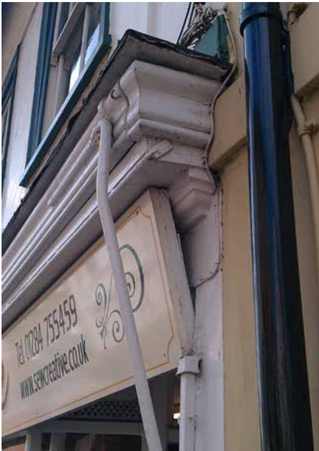
Detail of a closed traditional blind incorporated into the cornice above the fascia
