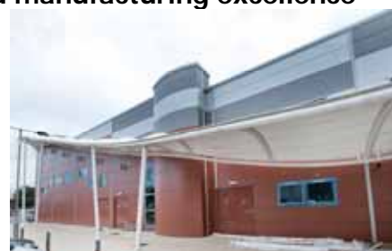
Haverhill Leisure Centre following a £5.2m refurbishment
