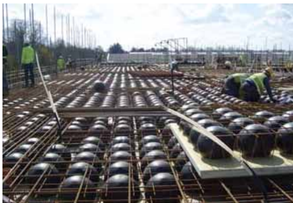
Bubble-deck floor construction
