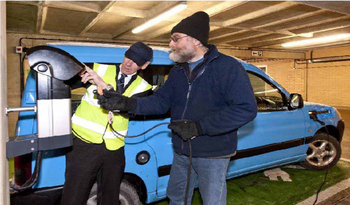
Parking spaces for electric cars, parkway multi-storey car park, Bury St Edmunds
