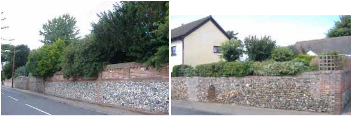
Photo 33: examples of flint walls
