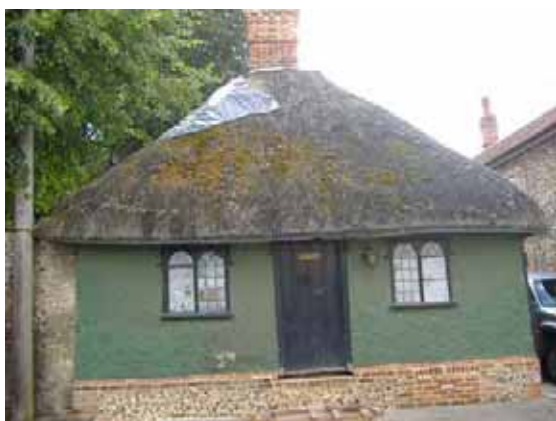
Photo 27: Early 19 th century former lodge to Stayer Cottage
