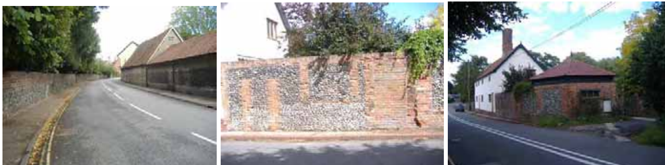
Photo 24: Buildings and walls line the street along Bury Road
