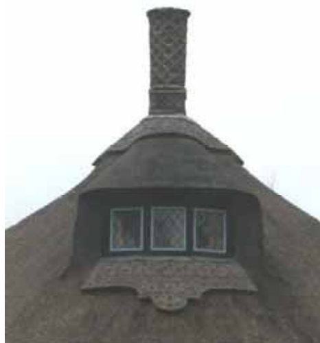
Photo 42: chimney and dormer of the Round House
