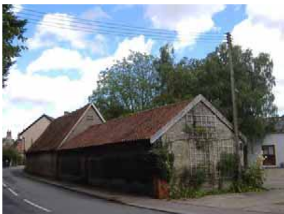
Photo 22: farm buildings in Bury Road
