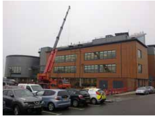
Installing solar panels at West Suffolk House, Bury St Edmunds
