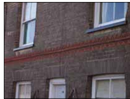
Victorian facades detailing (over timber frame) High Street
