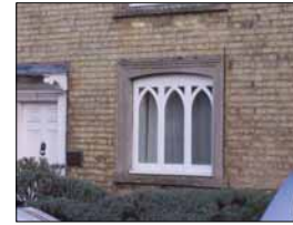
Gothic-Georgian windows - brick and stonework Queen Street
