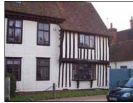
Timber frame, pargetting and leaded windows Nethergate Street
