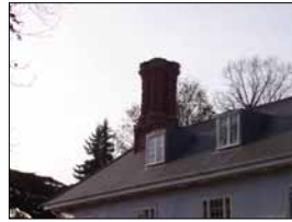
Decorative chimney and eaves detailing Cliftons, Nethergate Street
