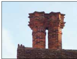
Highly decorative brick detailing Nethergate Street
