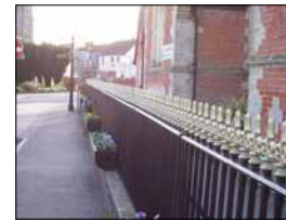
Signs and railings The Old School, Callis Street
